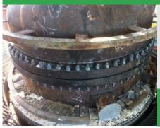
OMV Petrom Romania site required our assistance to install a critical gasket during a major shutdown. Our engineer supervised the entire installation of a specially designed Thermiculite® Kammprofile on the main reactor flange, resulting in a leak free start up on a critical vessel during a major shutdown, which enabled the site to meet industry best practice according to ASME PCC-1-2013.
